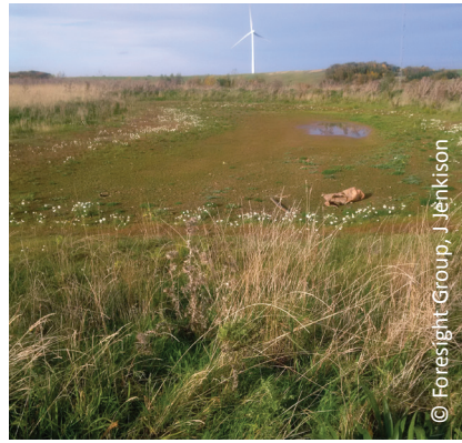
Balancing ponds are both an effective drainage management method that fill during high rainfall and gradually recede during dry weather periods whilst at the same time providing diverse habitats.
