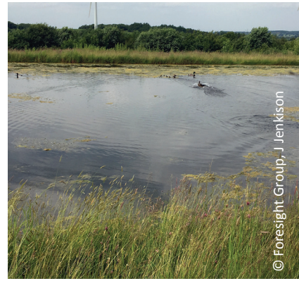
Balancing ponds are both an effective drainage management method that fill during high rainfall and gradually recede during dry weather periods whilst at the same time providing diverse habitats.
