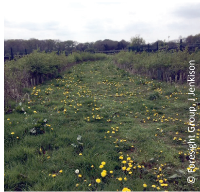
In this instance an existing public footpath in a natural depression was prone to flooding and the solution of slight levelling and planting dense hedgerows along either side of the route has resulted in hedge plant roots absorbing excess water flowing from higher ground and allowing the public footpath route to be rehabilitated as a wildflower meadow that is comfortable to traverse.
